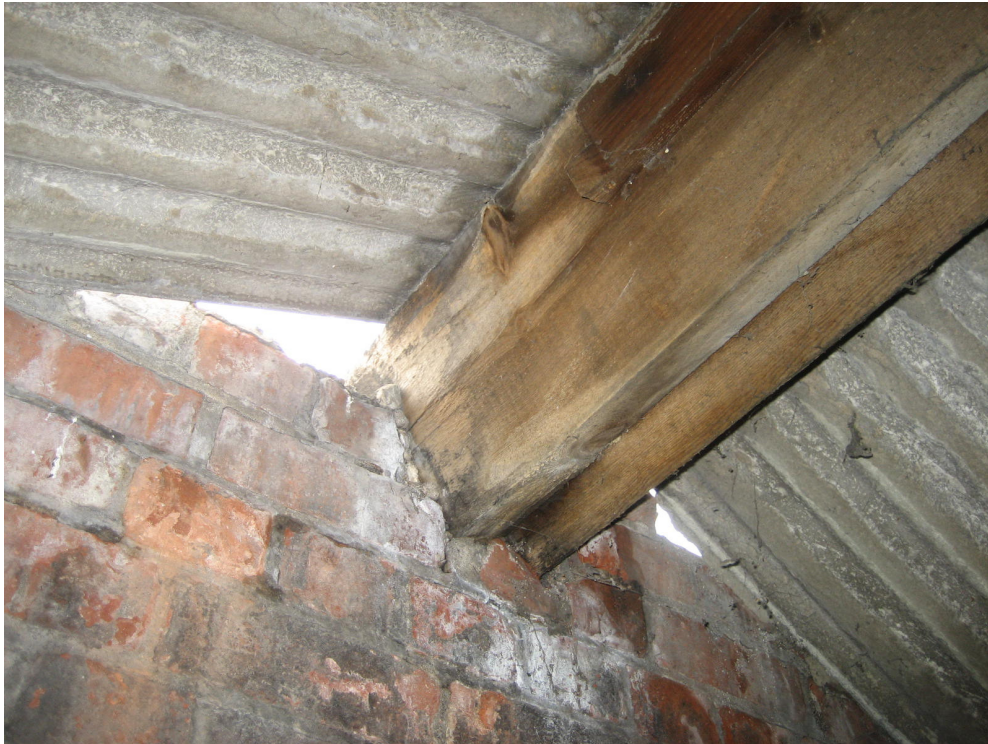
Photograph 49 Purlin bearing into wall above Piccadilly Entrance
