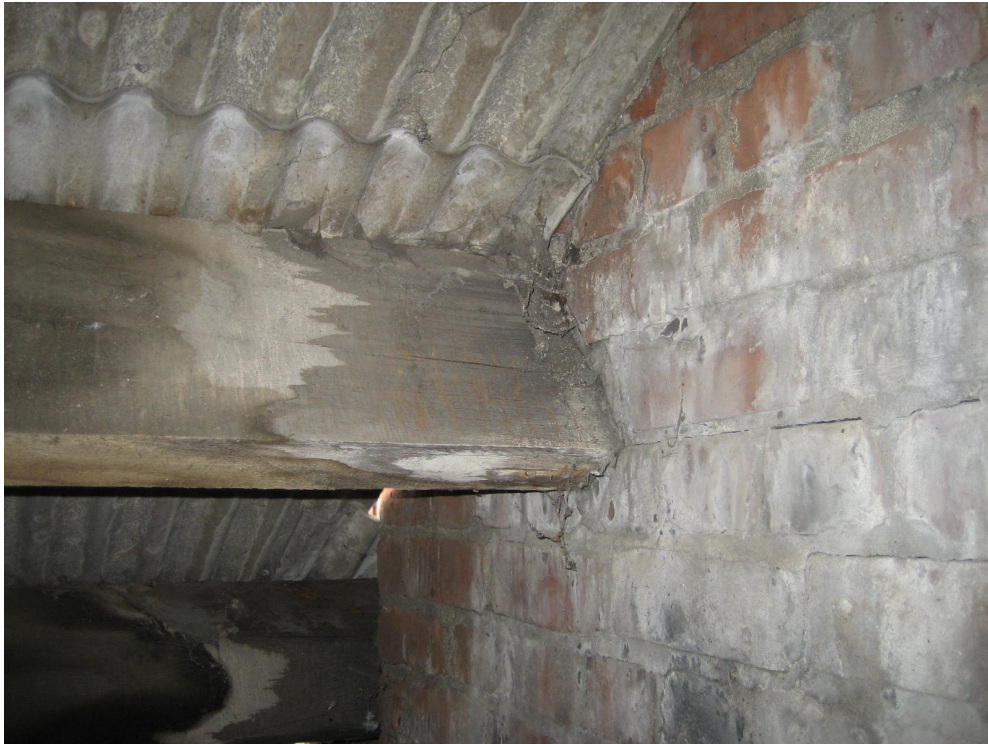
Photograph 51 Purlin bearing into wall above Piccadilly Entrance
