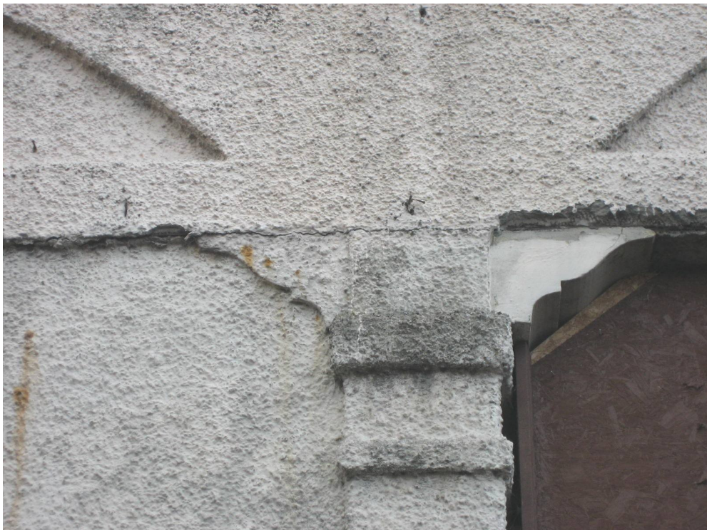
Photograph 26 Part North West Elevation
