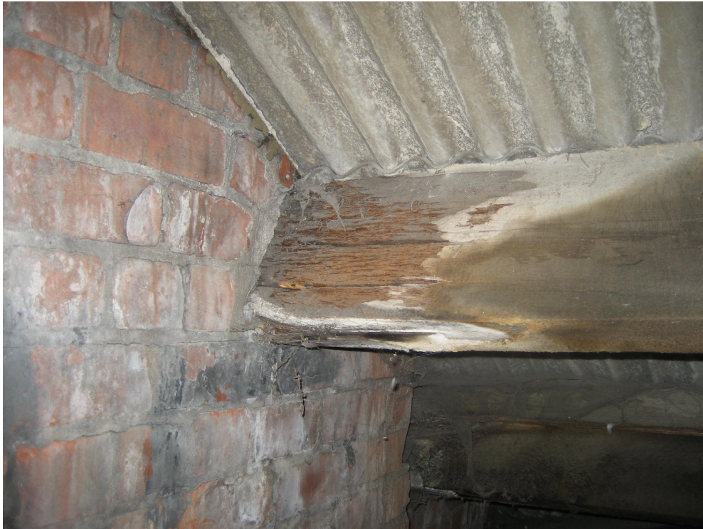
Photograph 47 Purlin bearing into wall above Piccadilly Entrance
