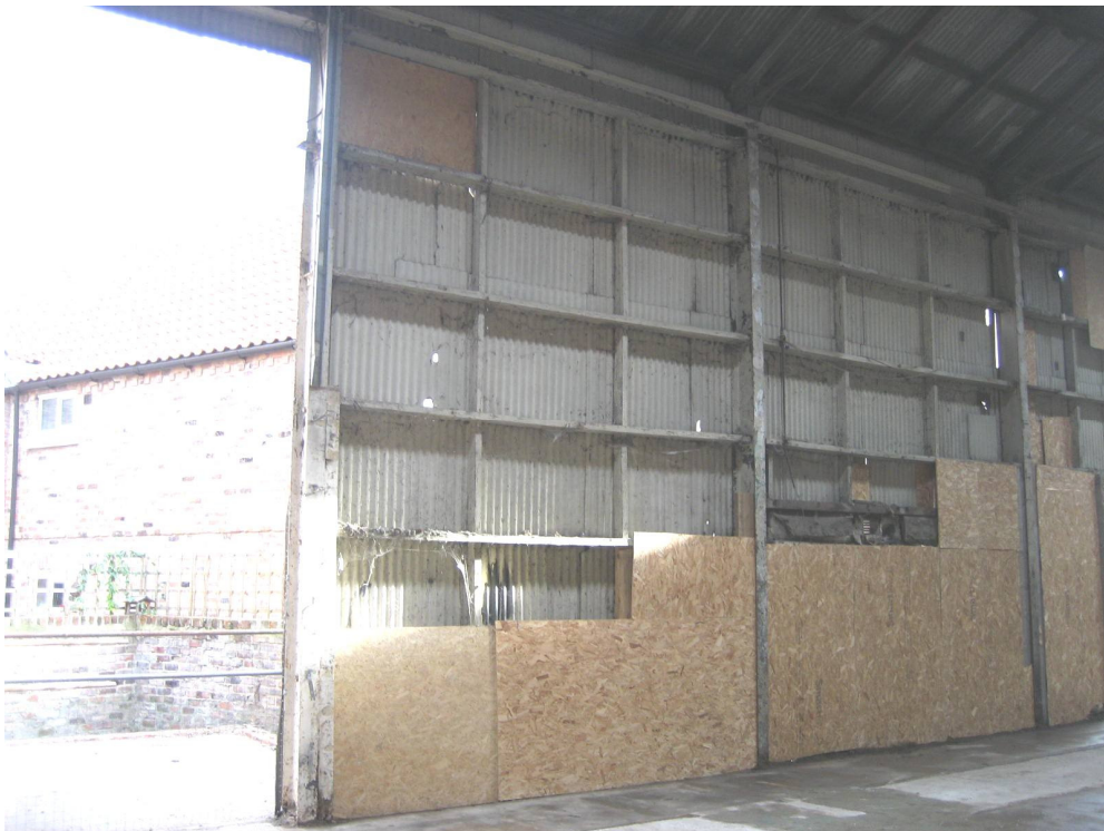
Photograph 40 Part view on rear elevation
