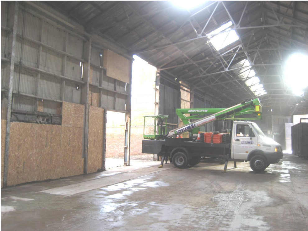
Photograph 41 Part view on rear elevation
