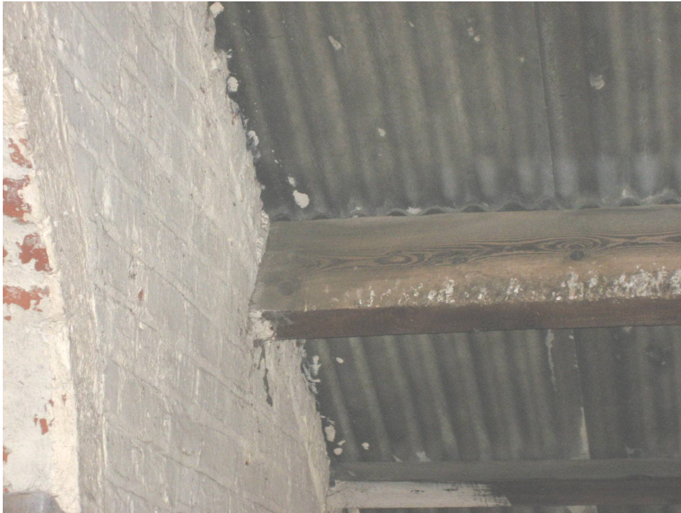
Photograph 55 Purlin bearing North West Entrance
