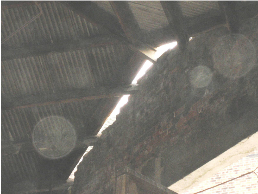
Photograph 35 Internal view above Dennis St. Entrance
