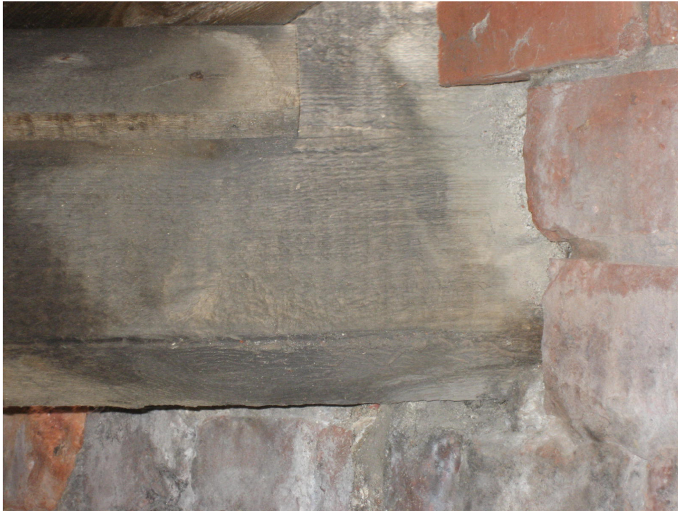
Photograph 57 Purlin bearing above Dennis St. Entrance
