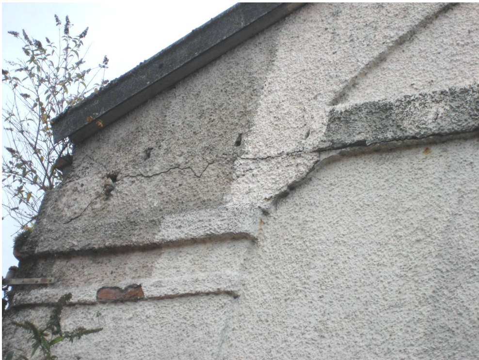
Photograph 28 Part North West Elevation
