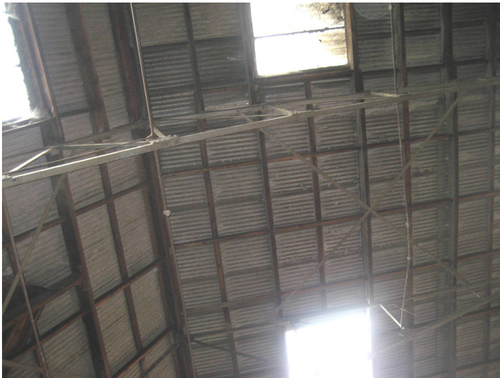
Photograph 53 Cross bracing in roof
