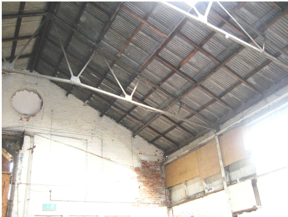
Photograph 38 Internal view towards North West Entrance
