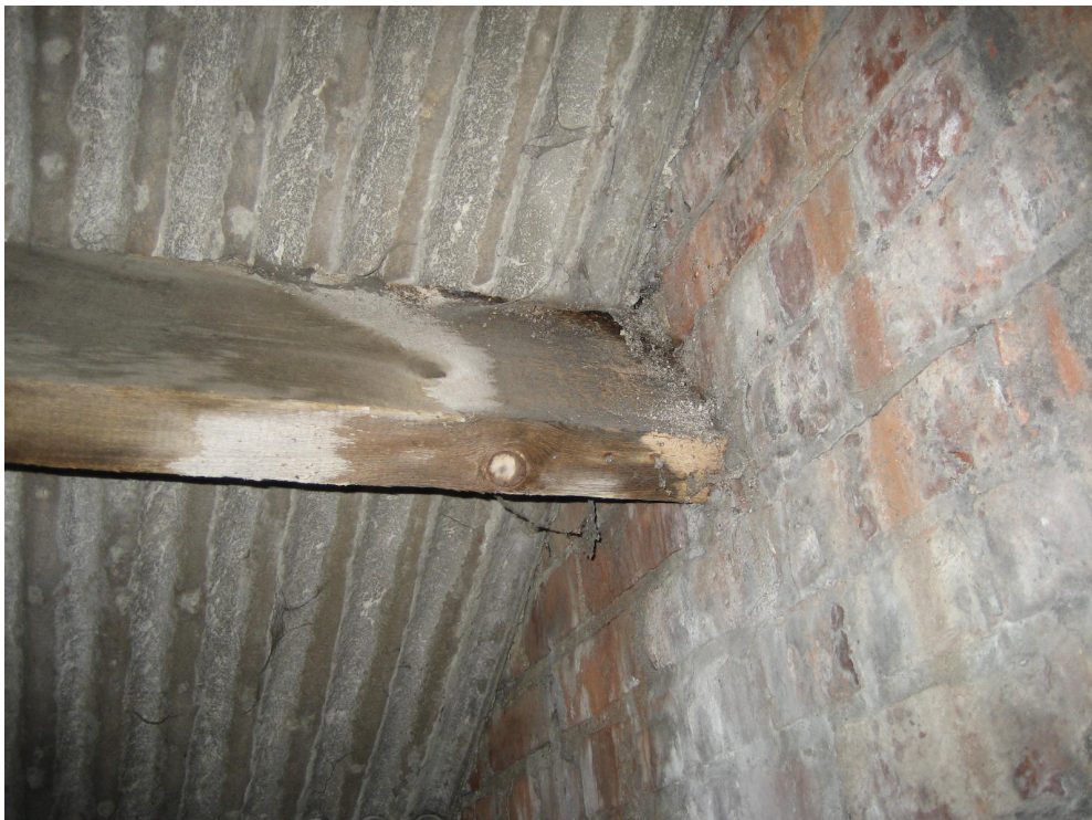
Photograph 50 Purlin bearing into wall above Piccadilly Entrance
