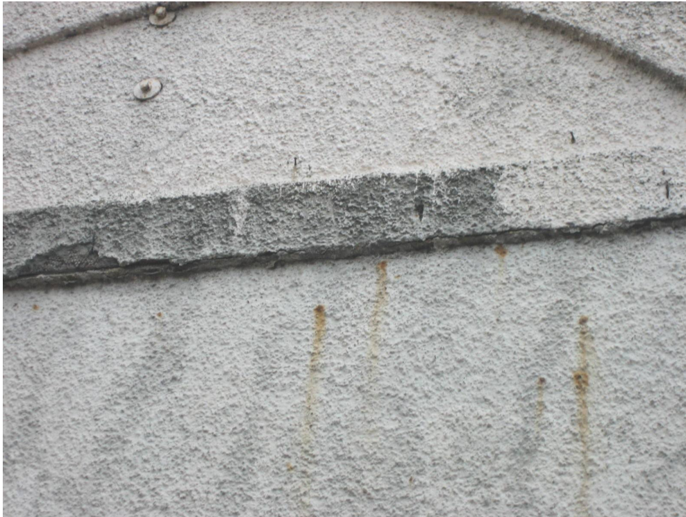
Photograph 27 Part North West Elevation
