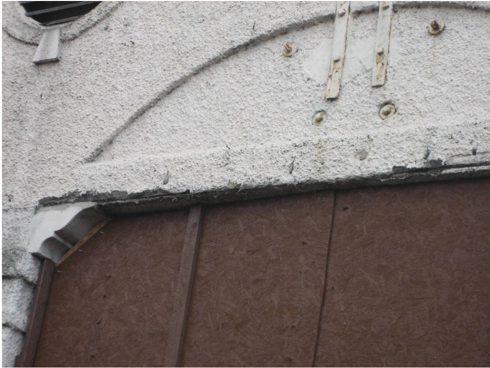
Photograph 25 Part North West Elevation
