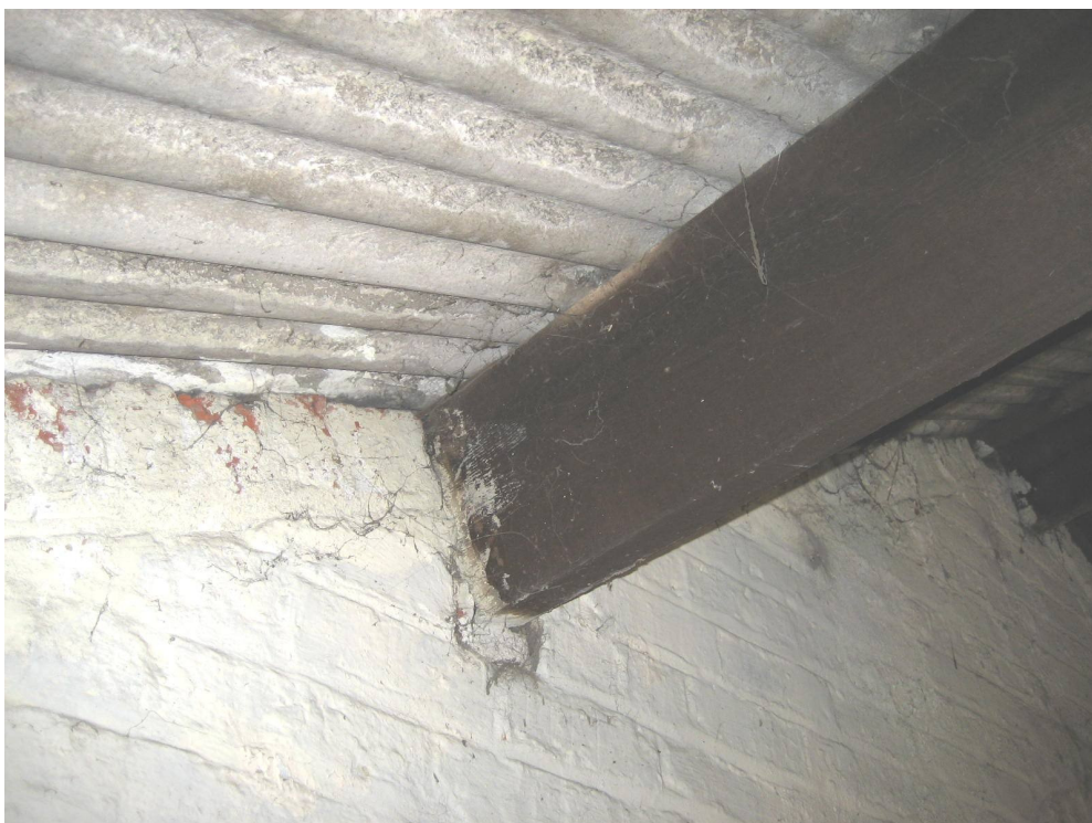
Photograph 54 Purlin bearing North West Entrance
