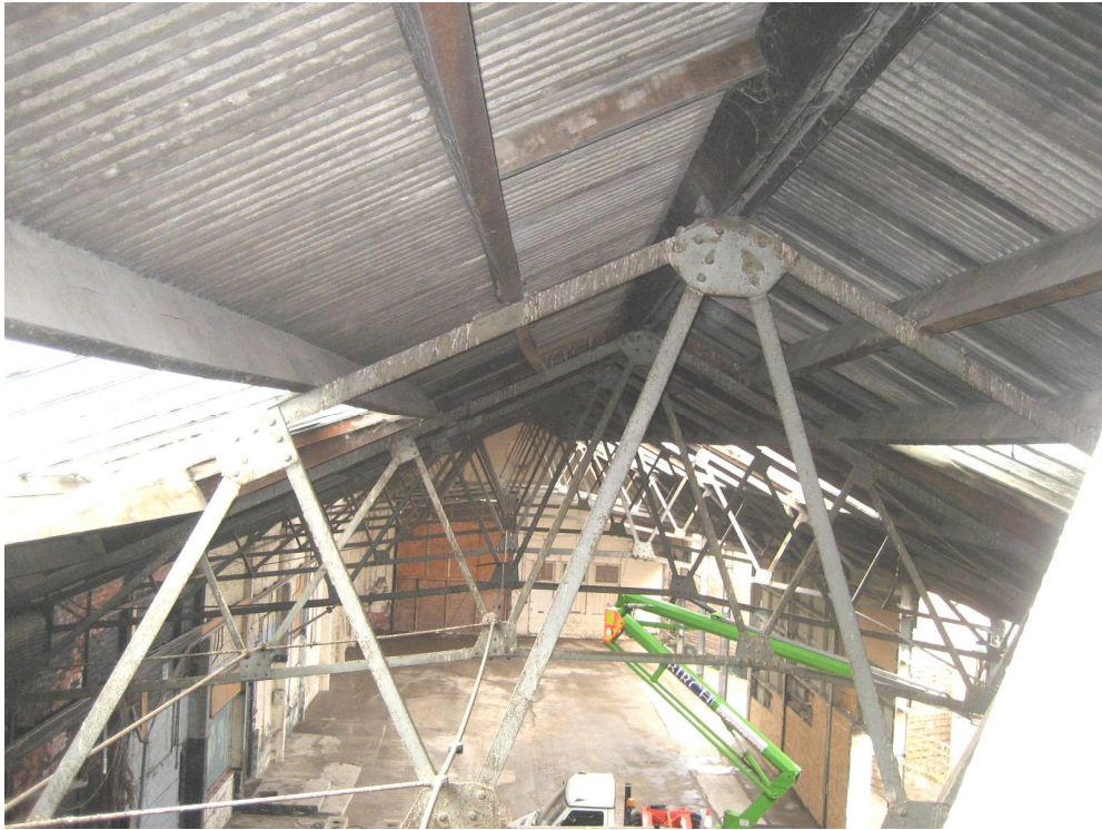
Photograph 45 High level internal view towards North West
