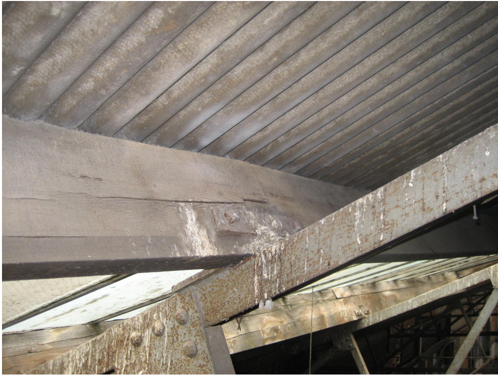
Photograph 43 Typical purlin connection
