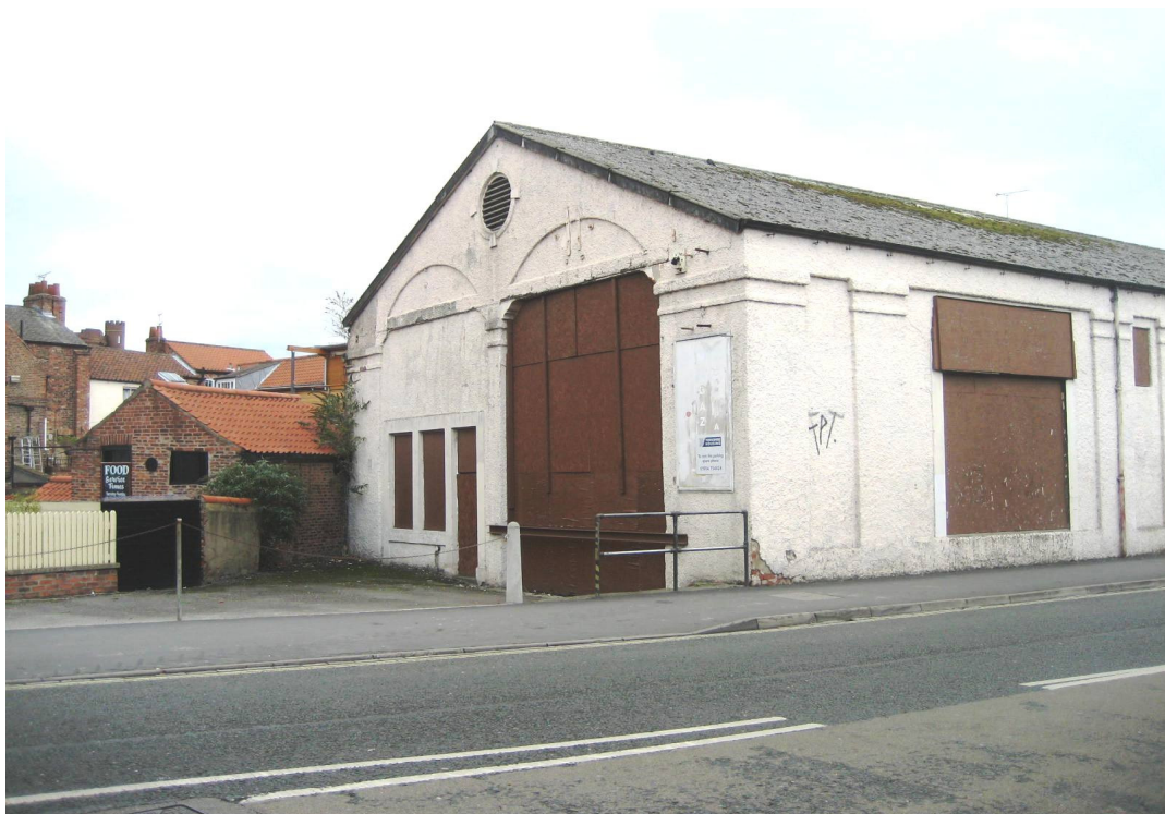
Photograph 4 North West Elevation
