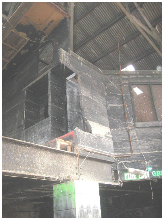
Photograph 42 partially demolished wall at Dennis St. end
