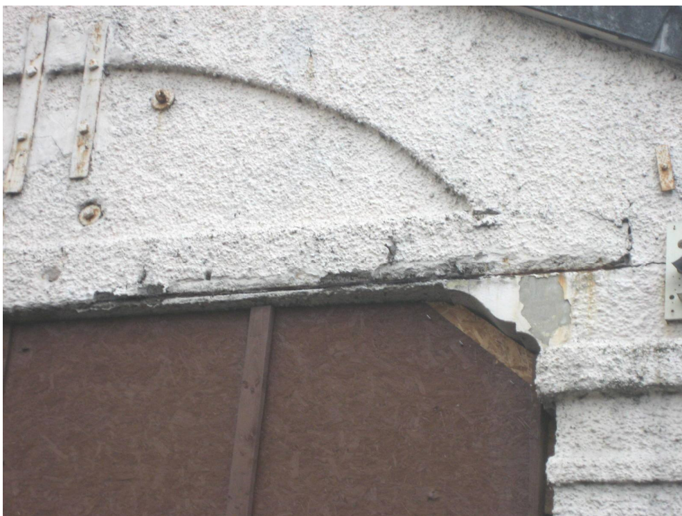
Photograph 24 Part North West Elevation
