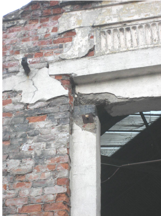
Photograph 31 Part Dennis Street Entrance Elevation
