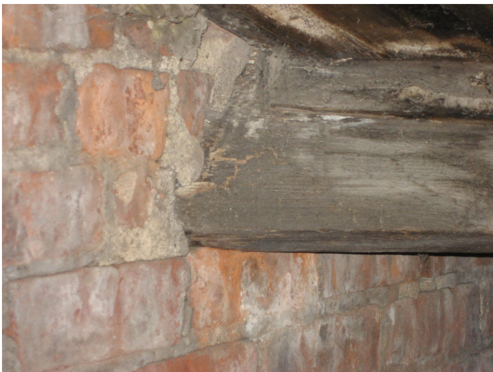
Photograph 56 Purlin bearing above Dennis St. Entrance
