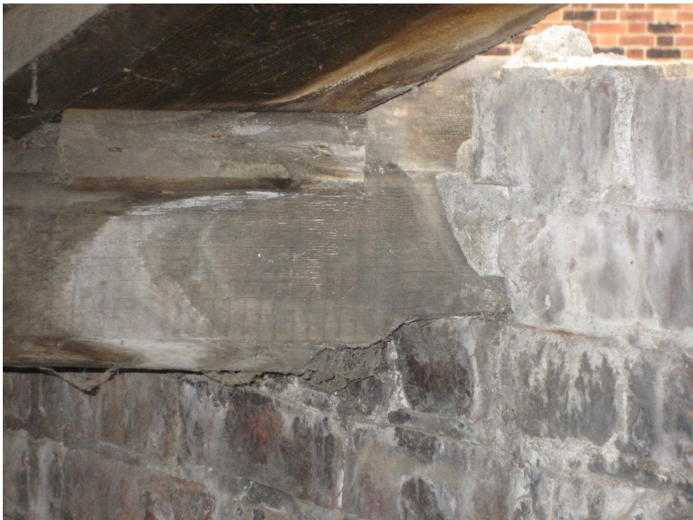
Photograph 58 Purlin bearing above Dennis St. Entrance
