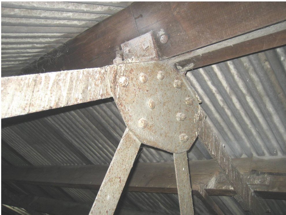
Photograph 44 Typical purlin connection
