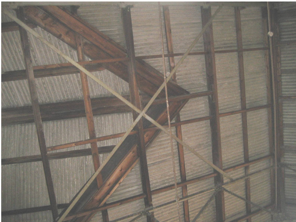
Photograph 52 Cross bracing in roof
