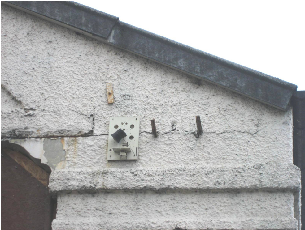
Photograph 23 Part North West Elevation
