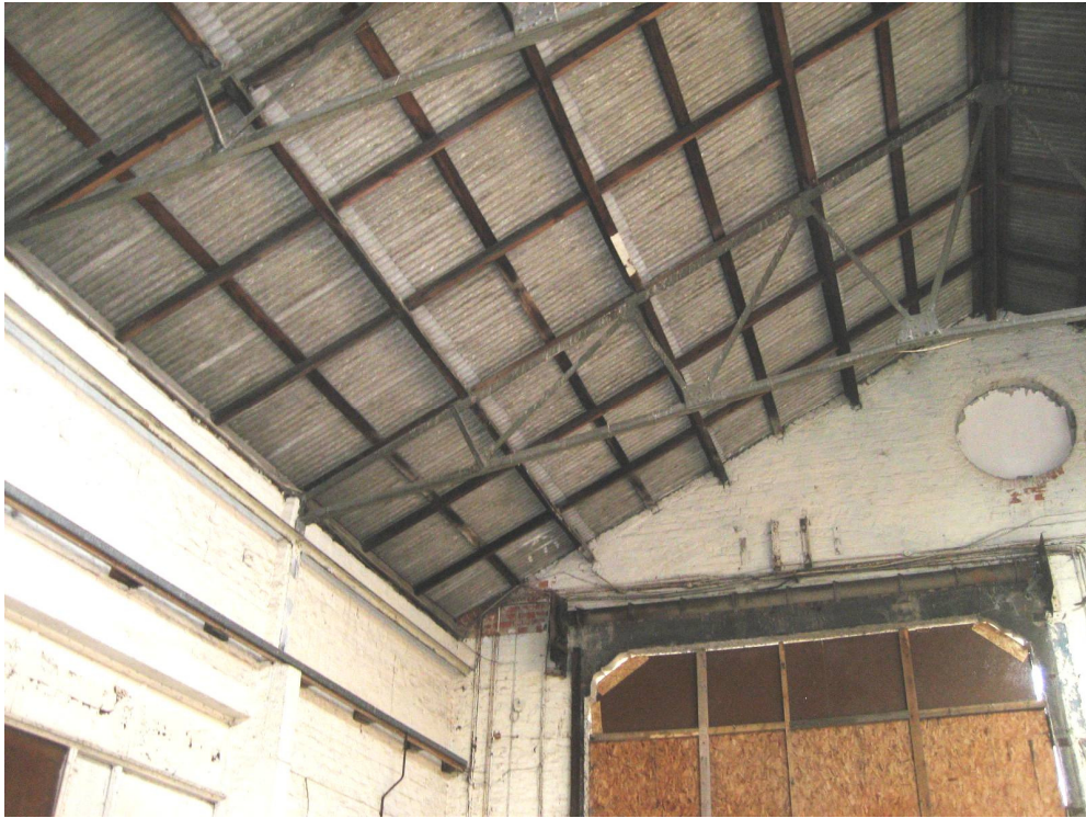
Photograph 37 Internal view towards North West Entrance
