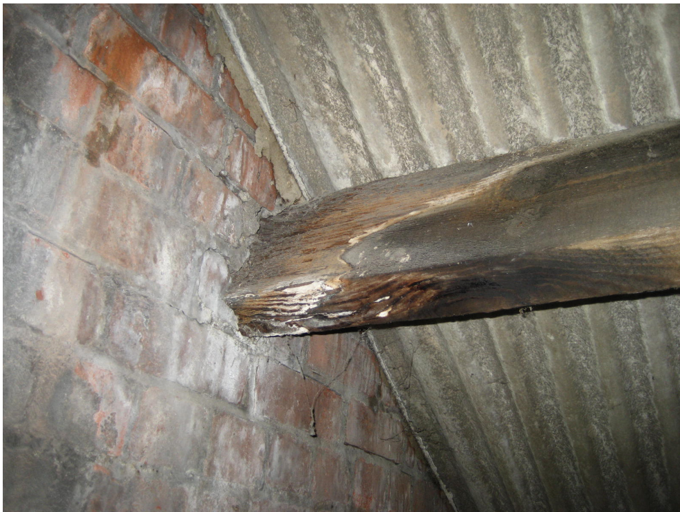
Photograph 48 Purlin bearing into wall above Piccadilly Entrance
