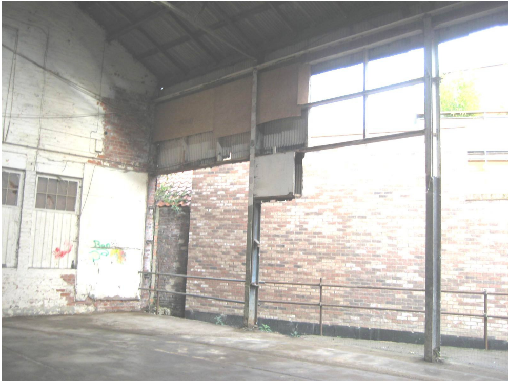
Photograph 39 Part view on rear elevation
